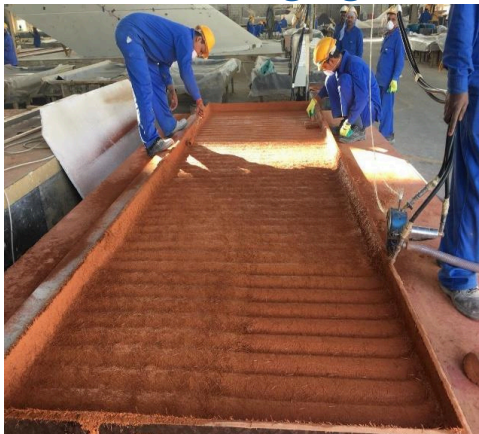
First Layer Compaction
